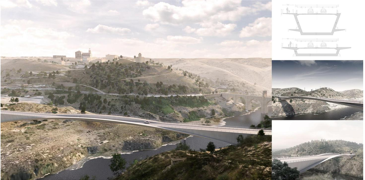
The solution we have called Ala is a bridge with a 3-span prestressed concrete lintel, with variable section, in which only the central span is visible.
